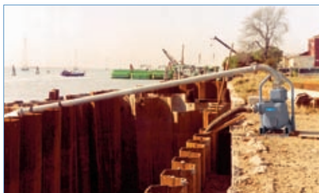
Construction site dewatering
