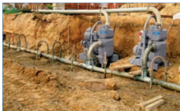
Wellpoint Vacuum dewatering
